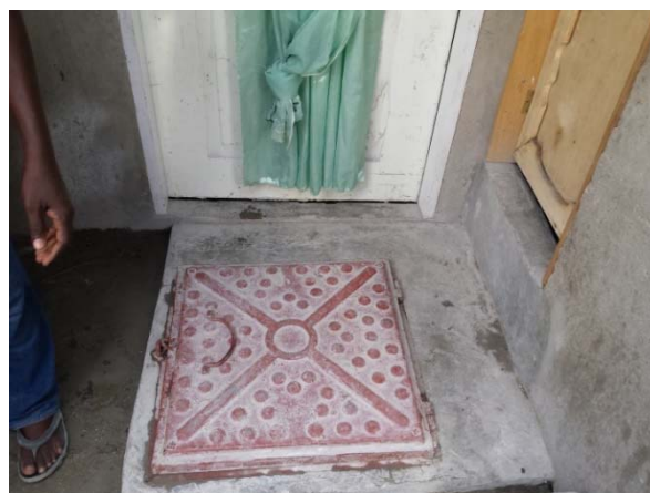
Picture 3. Location of septic tank cover in front of door with toilet to right (beneficiary has enclosed toilet area).
