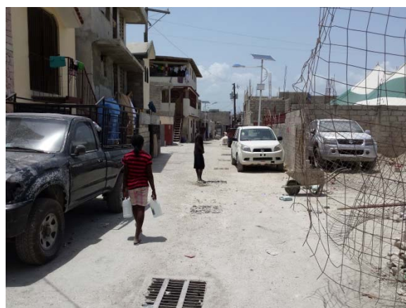
Picture 7. Paved pathways sloped to drainage below.
