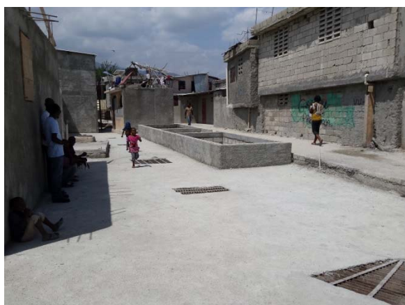
Picture 6. Open space adjacent to the canal.
