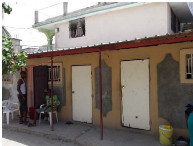
Picture 5. House that received materials and technical support for repair of roof.
