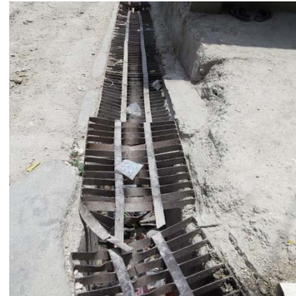
Picture 8. Metal grating used inferior materials on culverts in zones 3 and 5.
